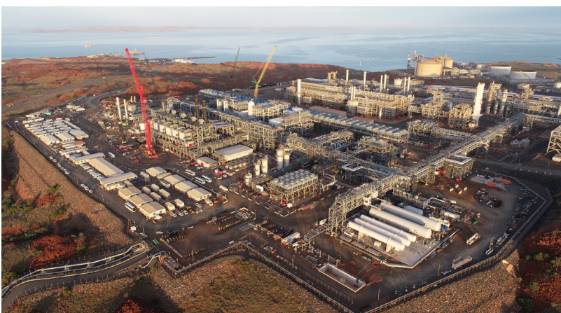
Figure 1 - Construction at Pluto Train 2 project site
