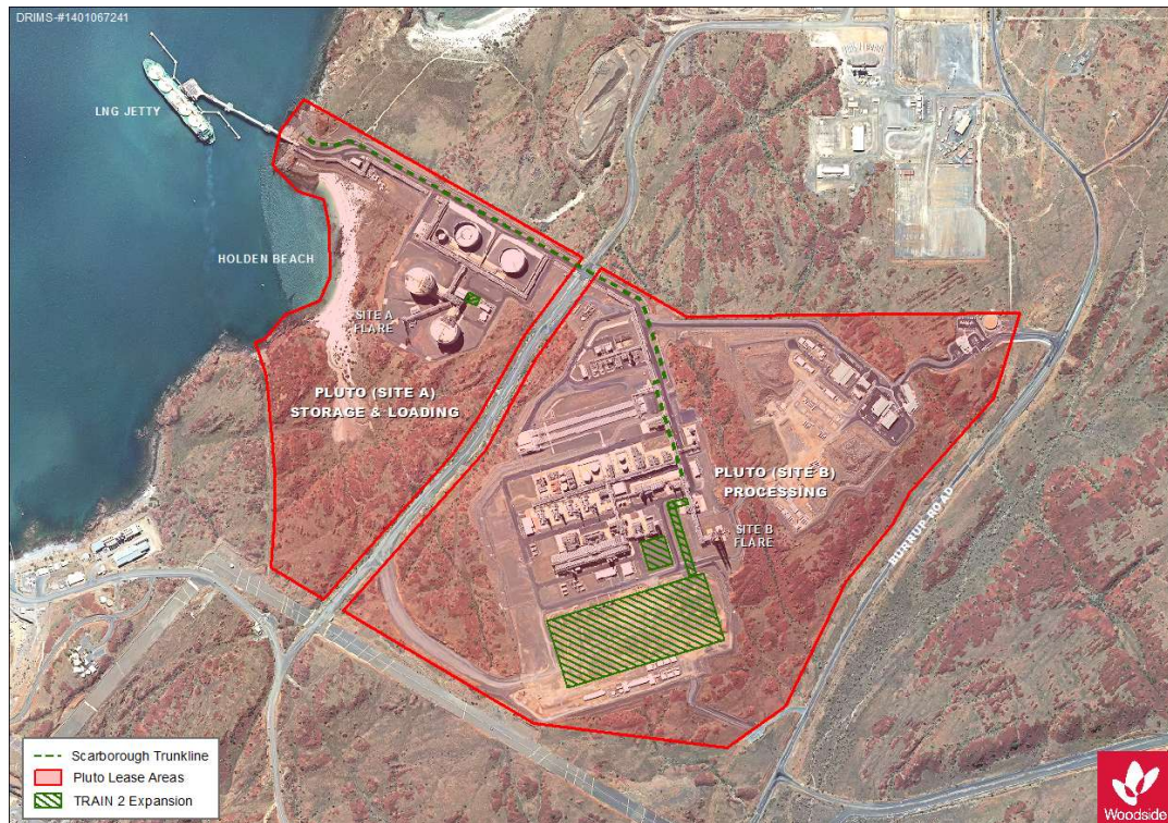
Figure 1 - Pluto LNG Site A and B on the Burrup Peninsula
