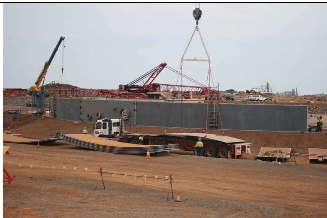
Plate 6: Condensate Tank outer shell construction, October 2008.
