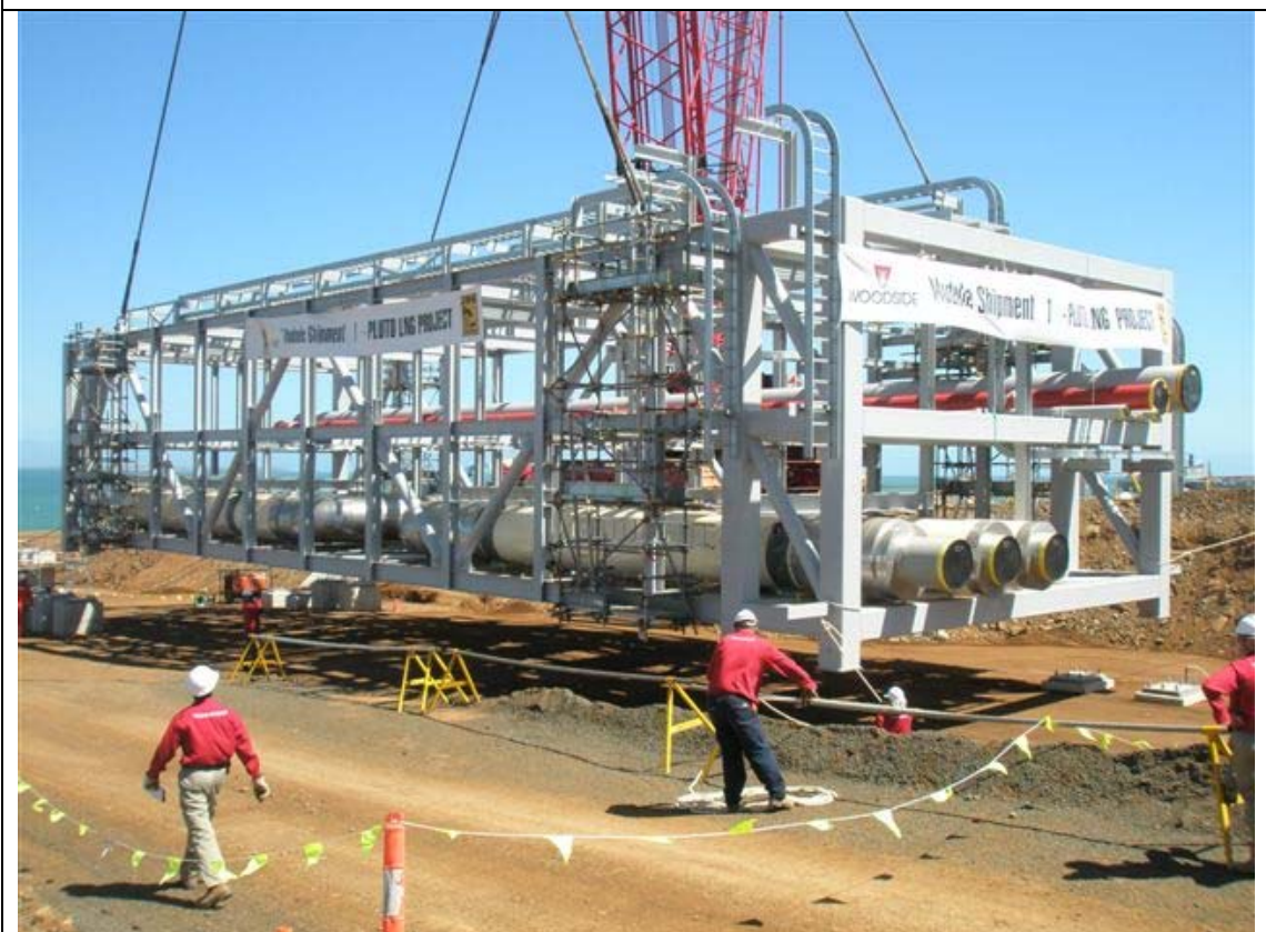
Plate 4: First preassembled pipe rack installed on Site A, November 2008.
