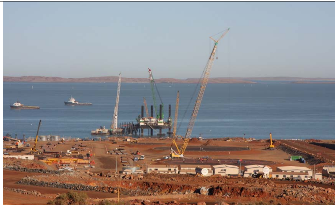
Plate 10: Site A construction, Jetty piling commenced after the completion of the Phase 1 dredging program, June 2008.
