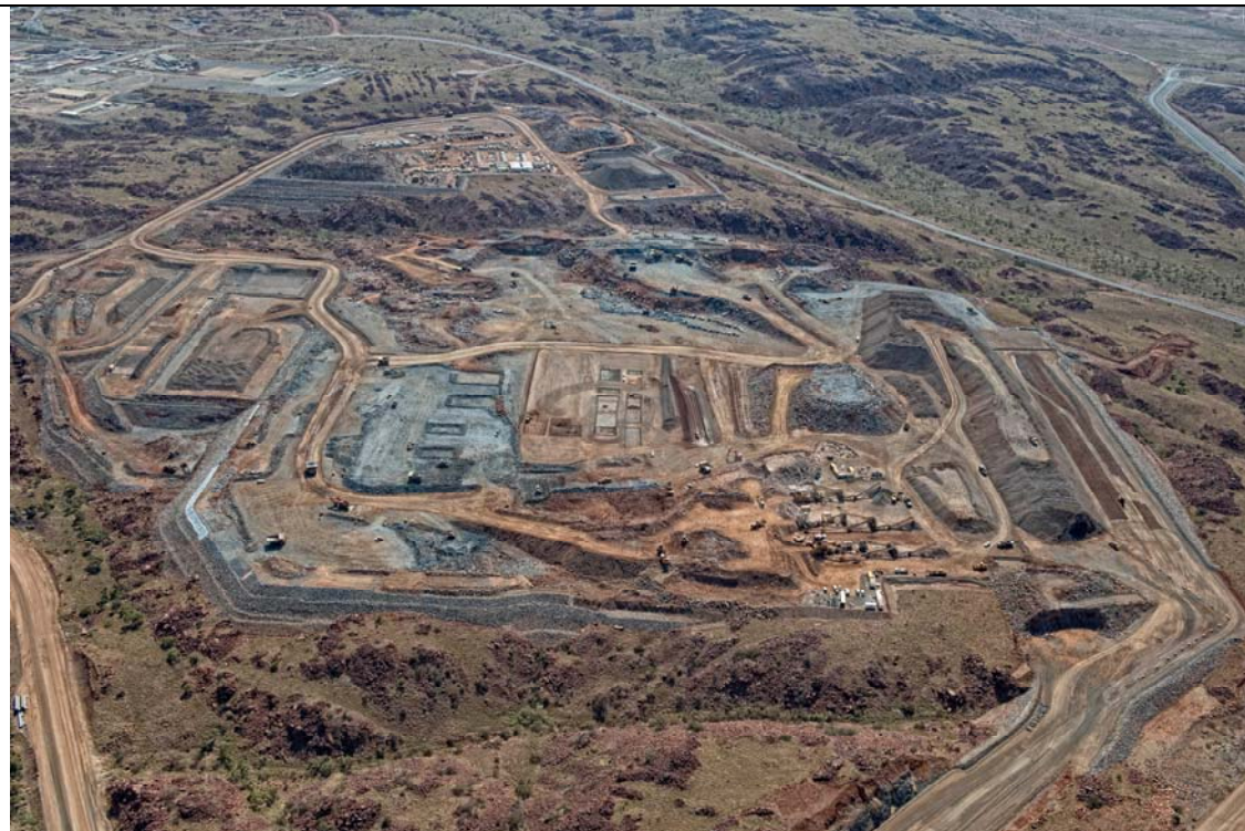
Plate 2: Site B Earthworks and pad preparation in preparation for train installation, 19 October 2008.
