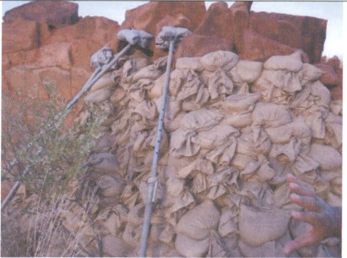
Plate 24. Heritage site protection measures. Sand bags are protecting the heritage item during site A preparation works.
