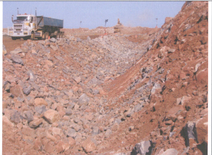
Plate 4. Drainage line beside major access roads to Site A.
