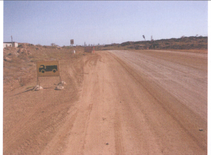
Plate 2. The designated access road or Haul Road.
