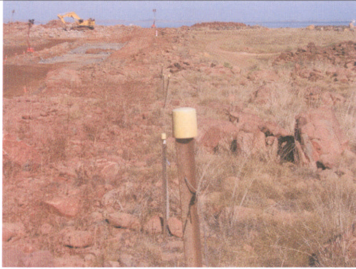
Plate 1. Disturbance boundary edge marked by yellow capped start pickets.
