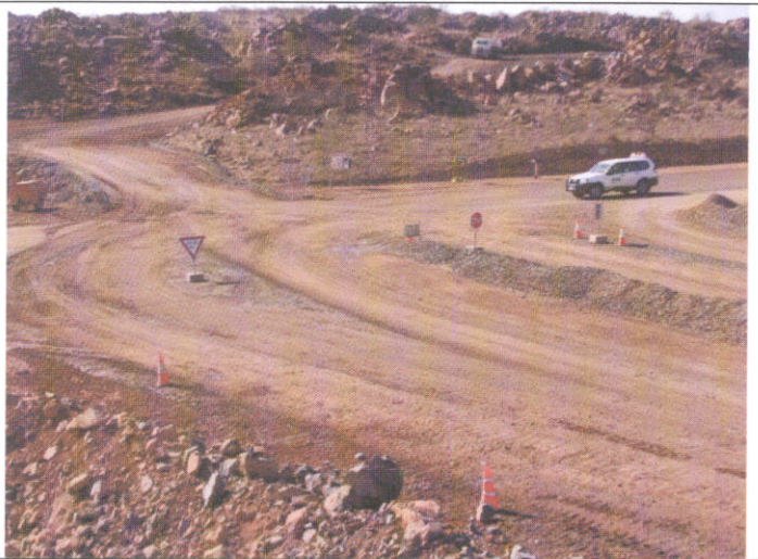
Plate 22. Site health and safety advisors are responsible for each traffic management activity such as this busy intersection of Site A and the Haul Road.
