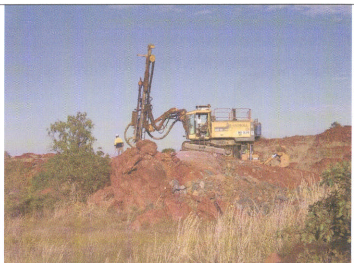
Plate 26. Drilling works prior to blasting activities.
