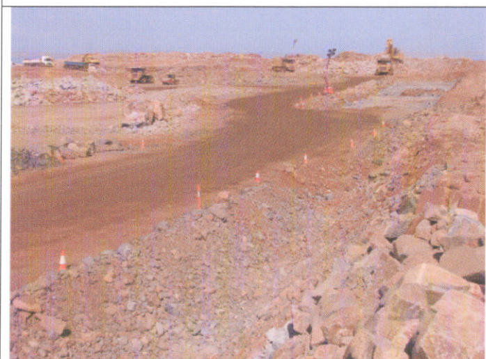
Plate 11. Traffic is kept to clearly delineated roads and tracks through the use of cones and bollards. Personnel are required to abide by a site speed limit of 20km/hr and 40km/hr on the Haul Rd.
