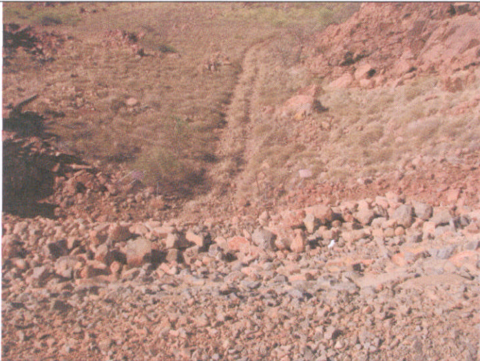
Plate 3. Geotextile lined drainage bund on the southern disturbance zone boundary.
