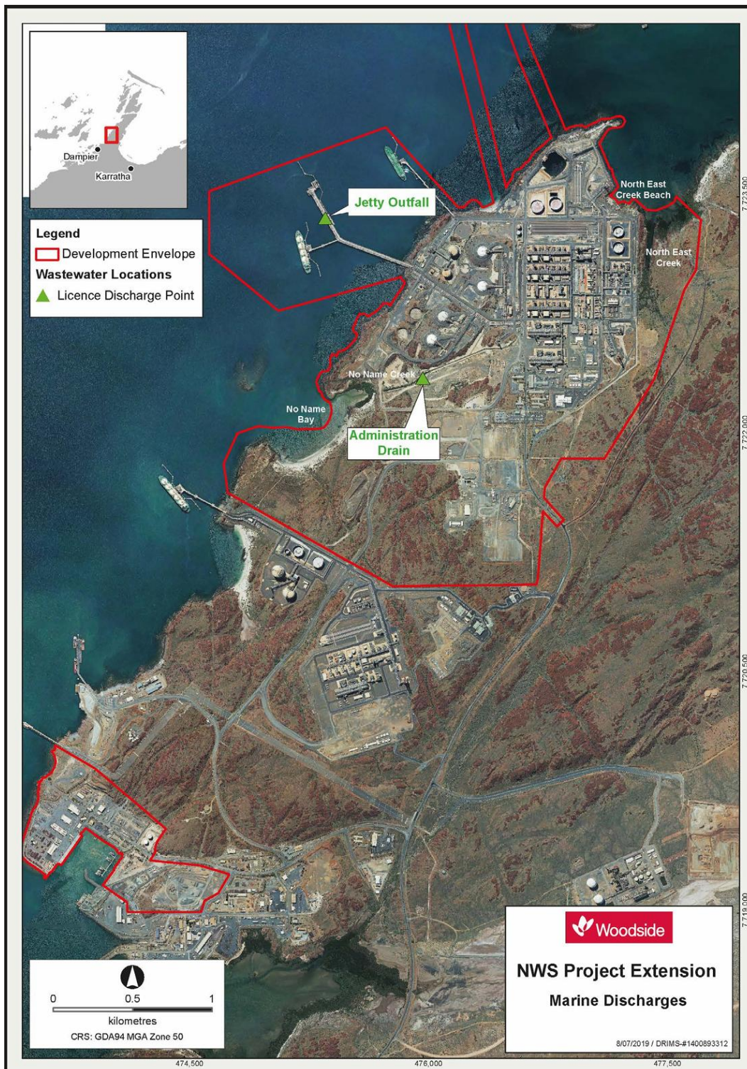
Figure 1-1 Wastewater discharge locations at Karratha Gas Plant (source: Woodside)
