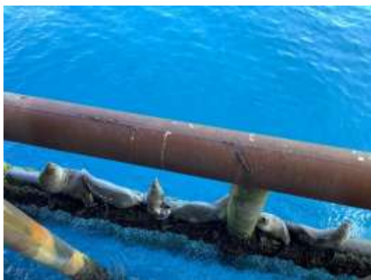
Seals observed on the Bream A steel piled jacket during the tracking survey
