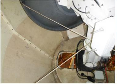
When a motor controller failed on board the Okha FPSO facility, a manual system involving a rope tied to the antenna bracket was set up to maintain the antenna tracking system until close collaboration with a vendor and speedy work paid dividends.
