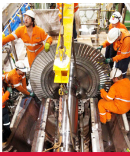
Top marks: Despite the many challenges, resilience and innovation helped deliver a best-in-class result in this year's turnaround. Left, contractor Hayden Harrison verifying calibration data. Right, installing a new turbine rotor.
