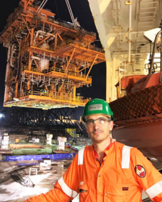
Water everywhere: Left, Henk-Jan Bakkenes of Heerema Marine Contractors was on deck as the water handling unit was lifted on to the Pluto platform (PLA); right, the 1700 tonne unit safely installed.
