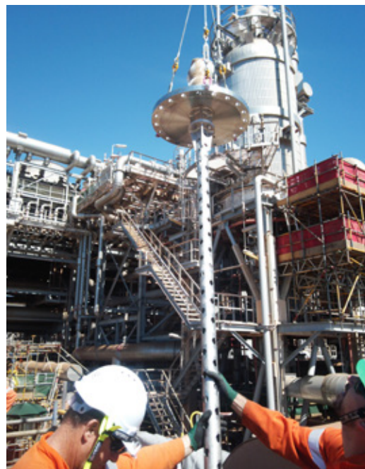
Job done: The Karratha Gas Plant (KGP) turnaround team celebrates the installation of the guided wave radar rod; right, the rod is inserted into the propane kettle at KGP’s Train 1.
