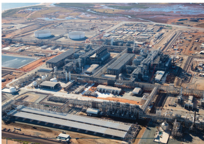
Wheatstone LNG is well advanced, with Train 1 nearing completion.
