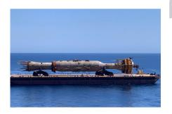
The Nganhurra RTM is a metal structure, about 83 metres long, on which Woodside previously moored an oil producing facility.
