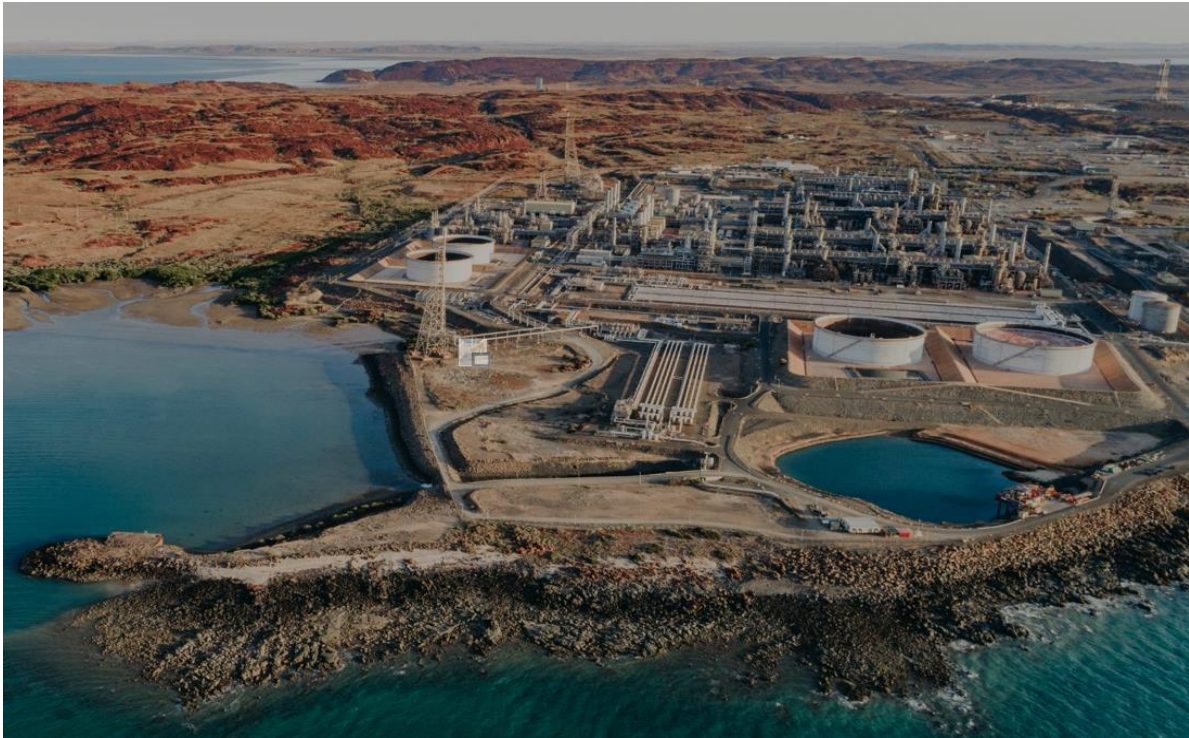
Figure 4.5: Karratha Gas Plant
